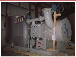
The Single Tower D<sub>2</sub>O Vapor Recovery Dryer removes heavy water vapor from reactor buildings. It consists of a tower filled with desiccant. Wet air is forced into the desiccant tower which absorbs water moisture. Dry air is re-circulated into the building. Desiccant is regenerated by passing hot air through it. Moisture is picked up by the hot air and condensed to recover heavy water.
