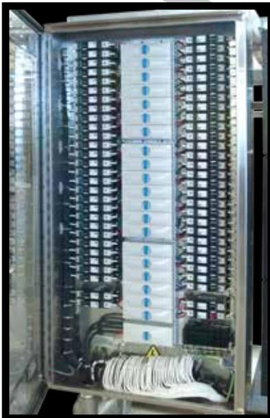
Power Distribution with Sealed Breakers
