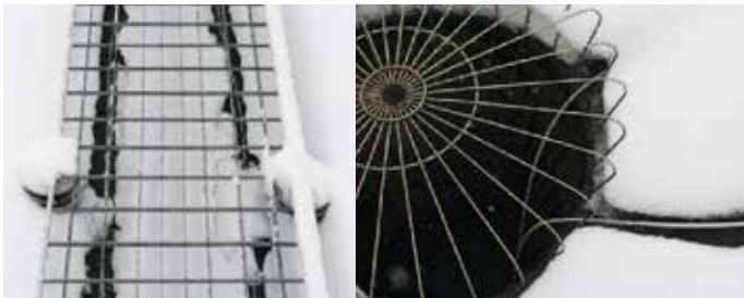
Of the 1,500 m<sup>2</sup> roof surface 1,000 m<sup>2</sup> is equipped with electric heating cables, at a spacing of 15 cm, resulting in a total length of 6,000 meters of heating cable, divided over 450 heating circuits.
