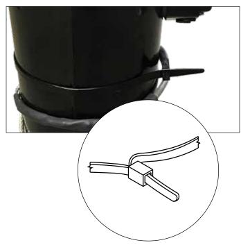
3. Connect CCH to power. A 240 Volt supply with 30mA earth leakage protection is mandatory.
