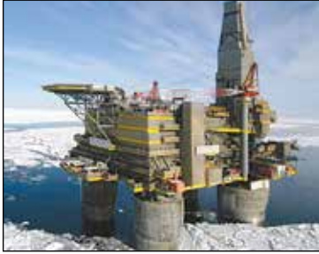
OFFSHORE OIL AND GAS PLATFORMS
