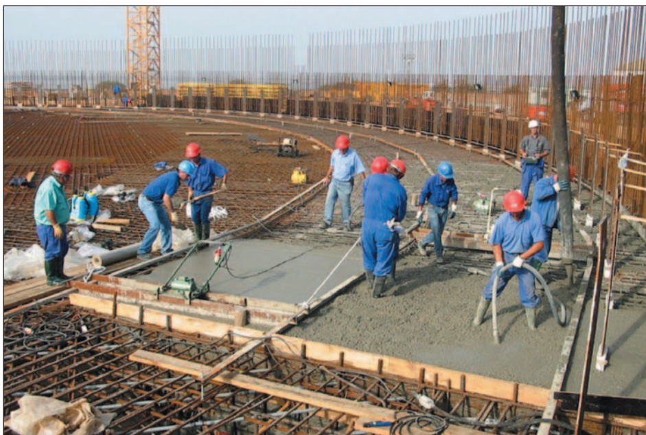
Fig. 8 Tank base under construction
