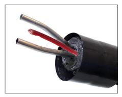
Place heat-shrink sleeve over end and prepare for final step.
