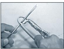
**Step 3:** Separate braid strands at overjacket and pull cable back through opening in braid.
