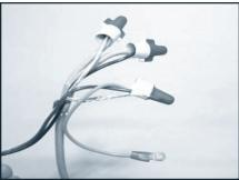
**Step 10:** The incoming power cable should also be provided with a drip-loop before it enters the enclosure. Connect the power conductors to the cable leads. Connect the incoming supply ground wire to the cable braid and to the green ground wire. Crimp the ring terminal to the other end of the green ground wire and then connect it to the grounding screw on the lock-ring.
