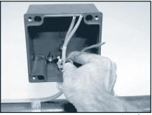
**Step 9:** Mount NEMA 4X junction box (not supplied) to support structure. The junction box should have one opening for incoming power and a 1" (25 mm) opening for the heating cable. For roof-and-gutter installations, mount box underneath roof eave if possible.
