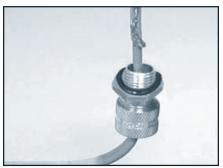
**Step 8:** Tighten the gland fitting to the cable such that the leading edge of the fitting is 1" (25 mm) back from the braid pigtail. Be careful to leave enough cable to easily reach the junction box without straining the cable.
