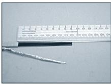
**Step 4:** Cut insulating jacket of cable back 3.5" (90 mm). Wind braid into a pigtail.
