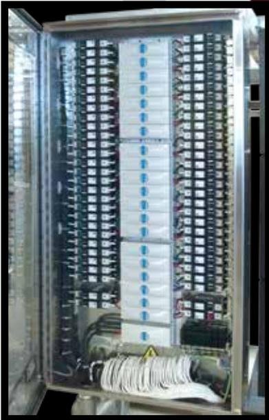
Power Distribution with Sealed Breakers
