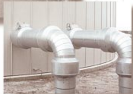
Protrusions from the tank are tightly fitted and sealed.
