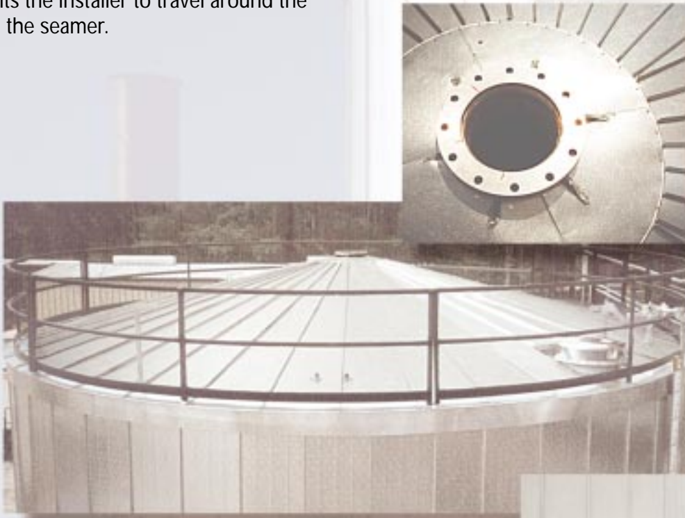
ThermaSeam panels installed radially on a tank roof provide a weatherproof surface.
