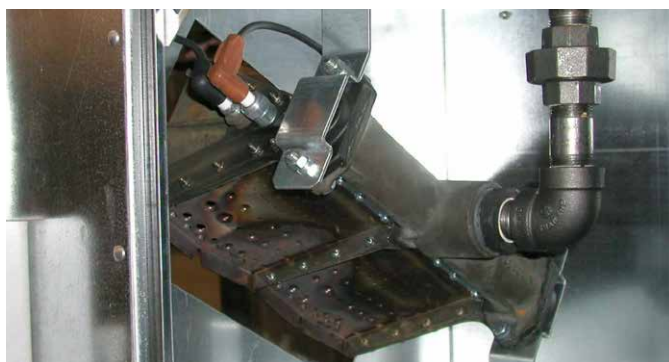
Figure 5 – Flame Rod and Spark Removal
