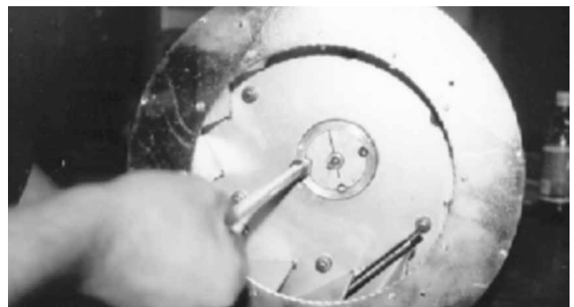
Figure 13 – Motor/Impeller Assembly Removal
