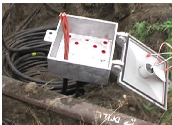
Figure 4 - Junction box mounted on pedestal in cable trench
