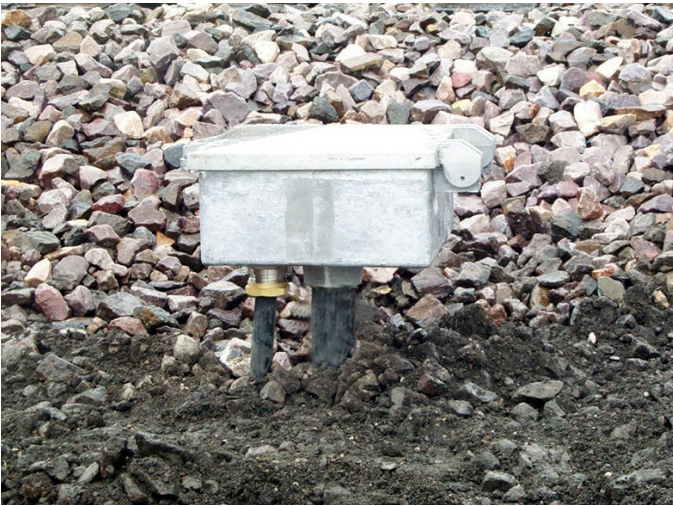
Figure 7 - Junction Box Installed
