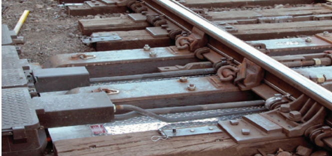
Figure 5 - Install clamps on rear heater every 2".
