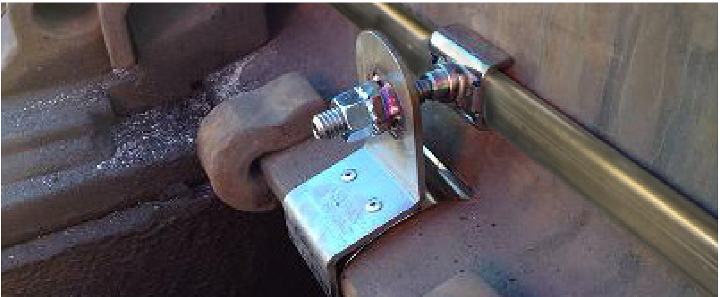
Figure 4 - Heater Installed with FRB clamp.(example only, clamp type varies depending on application)
