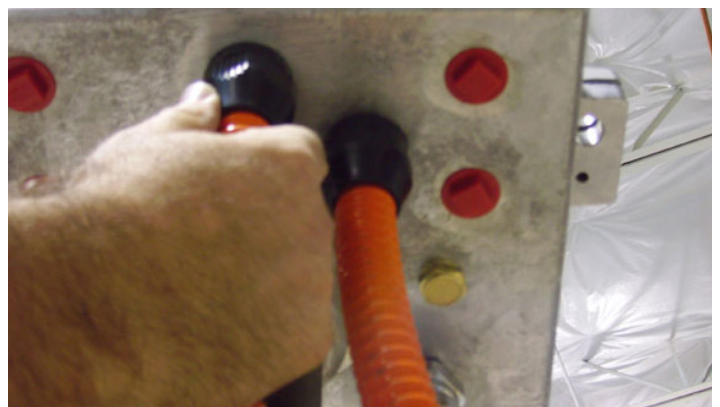
Figure 8 - Install as required with conduit or cable fitting
