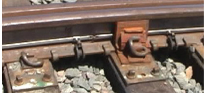
Figure 6 - Install the second heater from the rear of the switch so that the point of the rear heater meets the point of the front heater.
