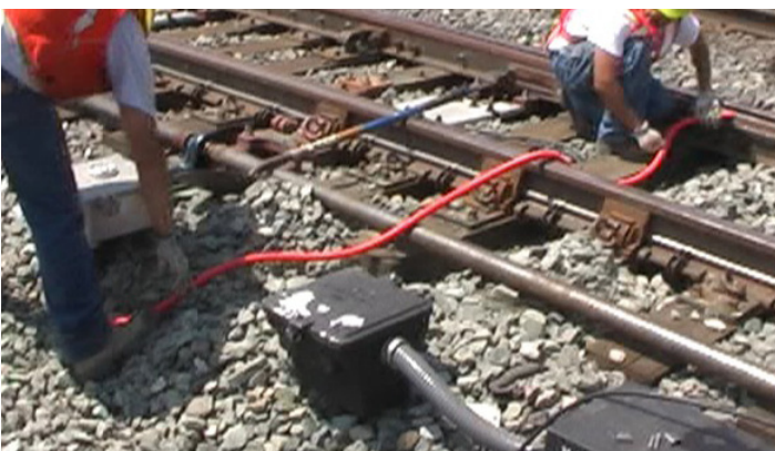
Figure 7 - Lead Wire shown installed with conduit.
