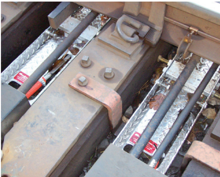
Figure 4 - Jack bolt Mount
