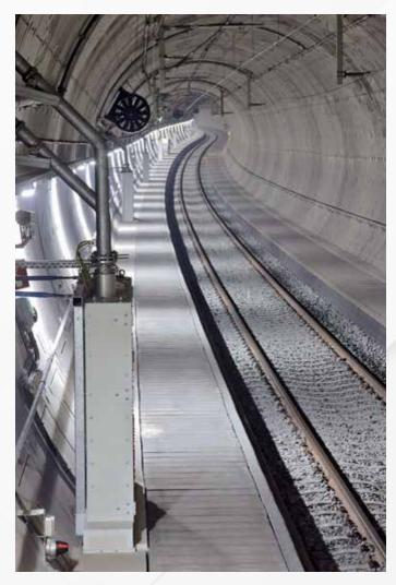
systems in the tunnels, between the hydrant and premix lines and the valve stations have been freeze protected with Thermon BSX self-regulating heating cables.
