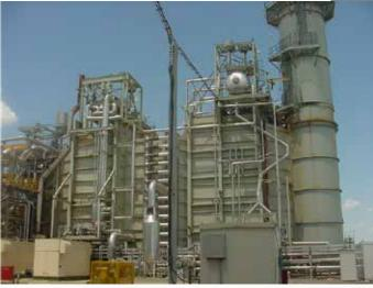
Typical HRSG units capture Combustion Turbine exhaust to generate steam. This is most often used for additional power generation.
