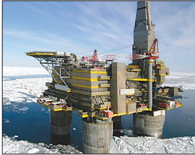
Offshore Oil and Gas Platforms
