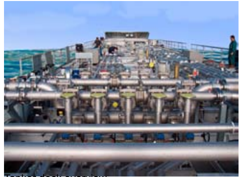
Tanker deck overview
