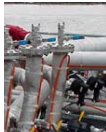
Tanker deck with heat tracing under construction
